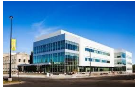
Figure 2. The Margaret Murie Life Science Building at UAF houses the Center's Admin Core, faculty offices/research labs, and the MRI suite of the Health and Metabolism Research Core (HaMR). Other Center facilities are located nearby on the UAF West Ridge.
