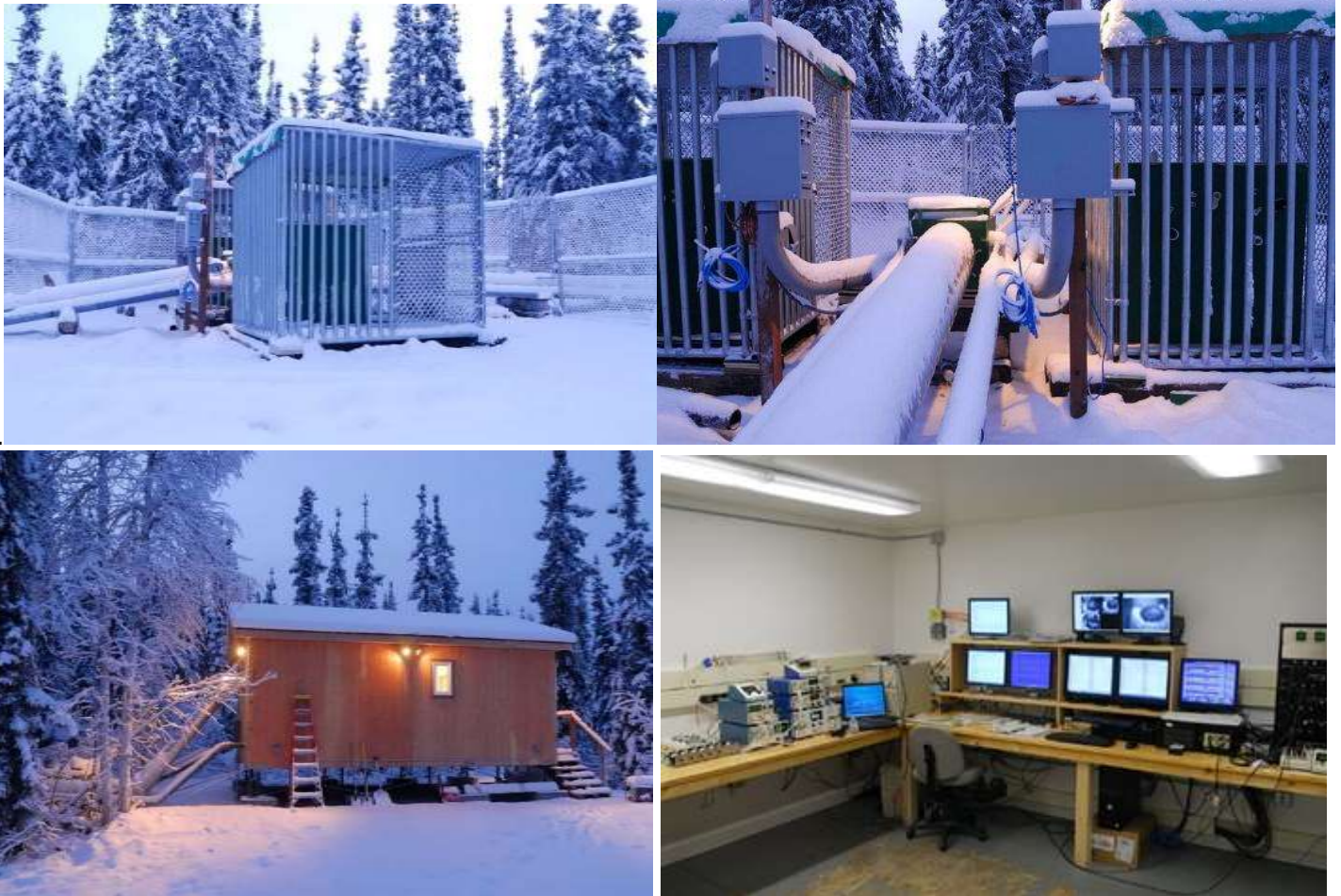
Bear Hibernation Facility (Figure 1) Hibernation facility showing two of the four cages, dens with instrumentation and instrument hut.
