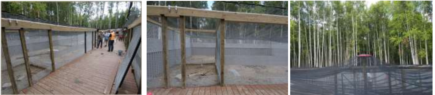
FIG. 2. AGS Breeding Facility alteration and renovation in progress, Summer 2020.
